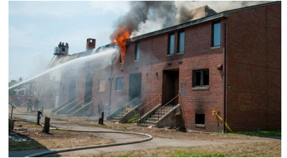
Applying water directly into the fire compartment as soon as possible results in the most effective means of suppressing the fire. 23
