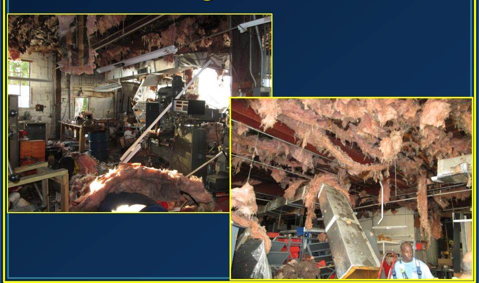
Large cylinders were thrown around the damaged area. In total there were 12 K/M cylinders found. 5 contained product.
